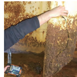
Port dock thickness measurement
