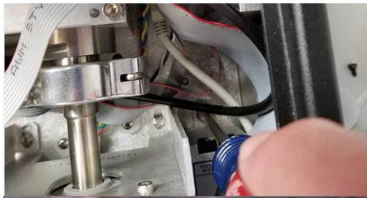
Figure 8.1.3.5-A Disconnecting Barometric Reference
